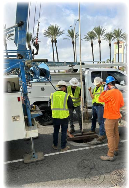
Rehabilitation Conducted on a Monitoring Well
